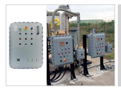
Heat exchangers and duct heaters are supplied with electrical control panels using Thyristor and PID thermoregulators for precision control. Additional instrumentation for other thermal and non-thermal control requirements can be
